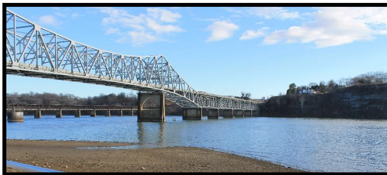
O'Neal Bridge near McFarland Park, Florence
