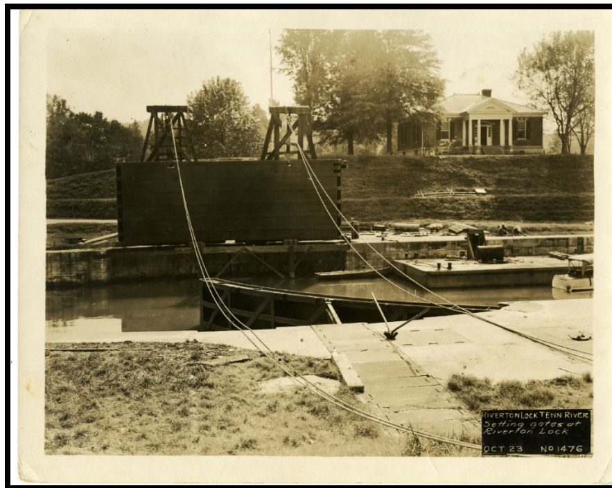
(The Colbert Shoals Canal Lock in Riverton, Alabama)
