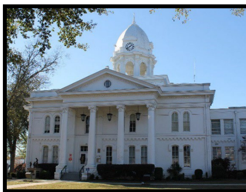
Colbert County Courthouse in Tuscumbia, Alabama
