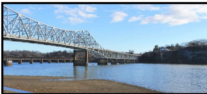
O'Neal Bridge near McFarland Park, Florence
